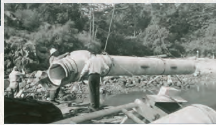
1980-015-258c Construction of Arbutus Outfall 1955
